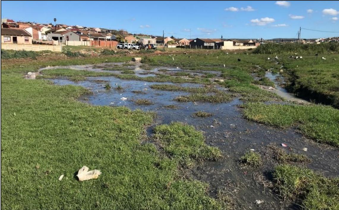
**Figure 3-40** A surcharging sewer manhole pictured centrally, and a newly incising channel pictured to the right located in CVB 3. The lateral tongues of the incising channel (heading towards the manhole) and the proximity of the point of incision to this surcharging manhole indicate that this manhole has been a large causal factor in the incision of this channel
