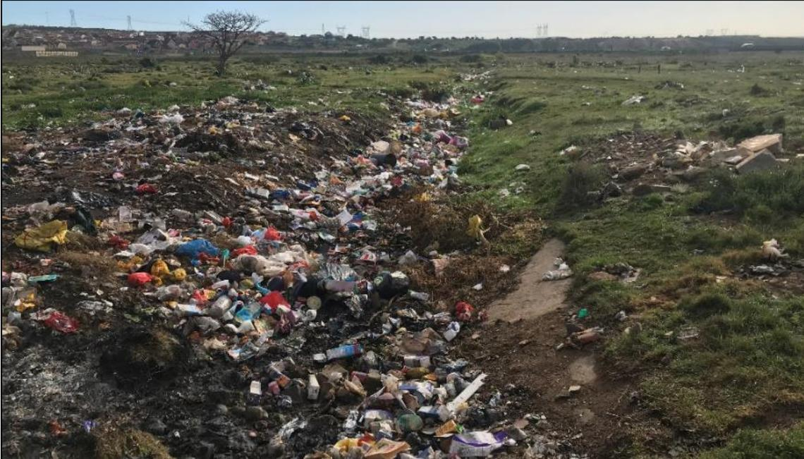
**Figure 3-36** One of the many stormwater canals that conveys stormflows into the Chatty River Wetlands. Many of these canals have been totally blocked by the litter and debris, causing them to overflow into inhabited areas, potentially posing a health risk to those living nearby. In addition, the canalised stormwater conduits that are not blocked were observed to, in some cases, have resulted in erosion and scour of the downstream wetland.
