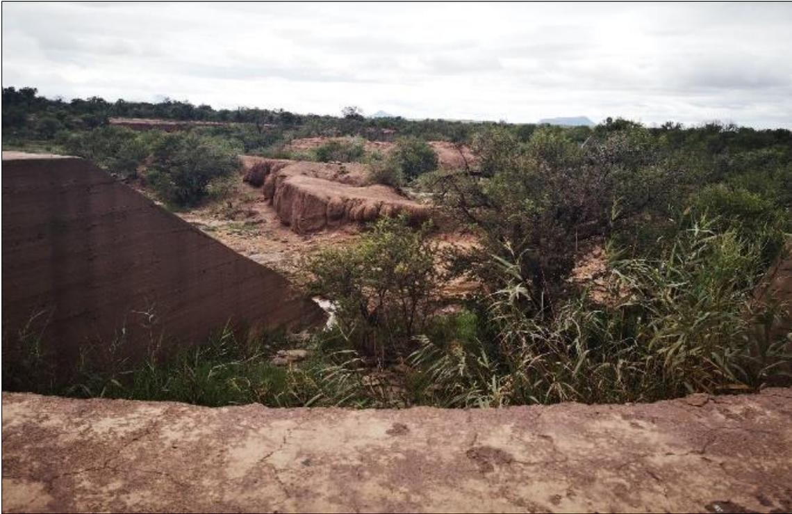
**Figure 3-50** View of the erosion gully downstream of a weir
