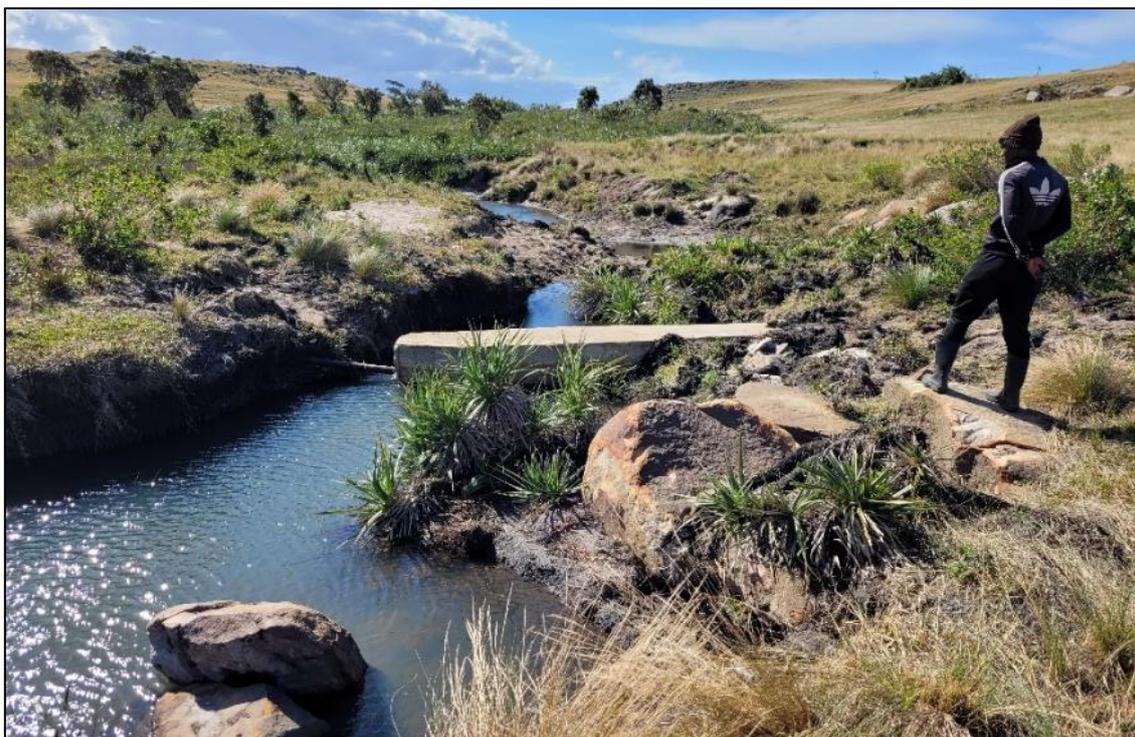
**Figure 3-115** Xolobeni wetland: Eroded palmiet wetland upstream of the water supply pipeline crossing point. Portions of the pipeline has been encased in concrete, however the channel has bypassed the concrete and has exposed portions of the pipeline
