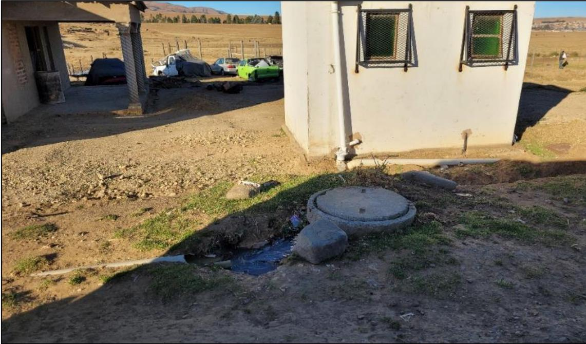
**Figure 3-92** Surcharging manhole with the sewage being directed towards the wetland
